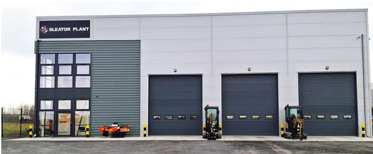
Sleator Plant's new Dublin depot.
